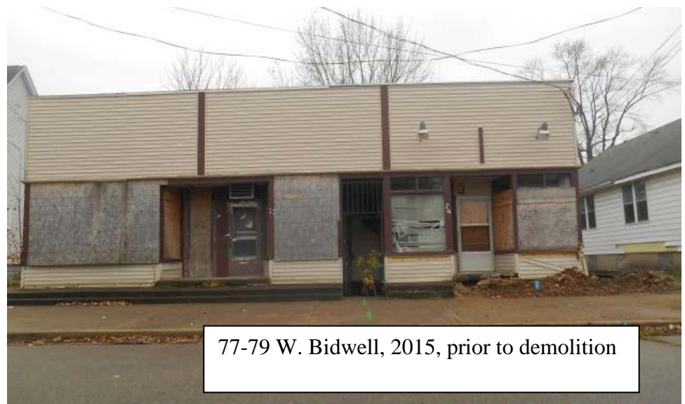
93 W. Bidwell, 2013, prior to demolition
